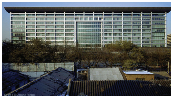
ICBC World Headquarters in Beijing.
